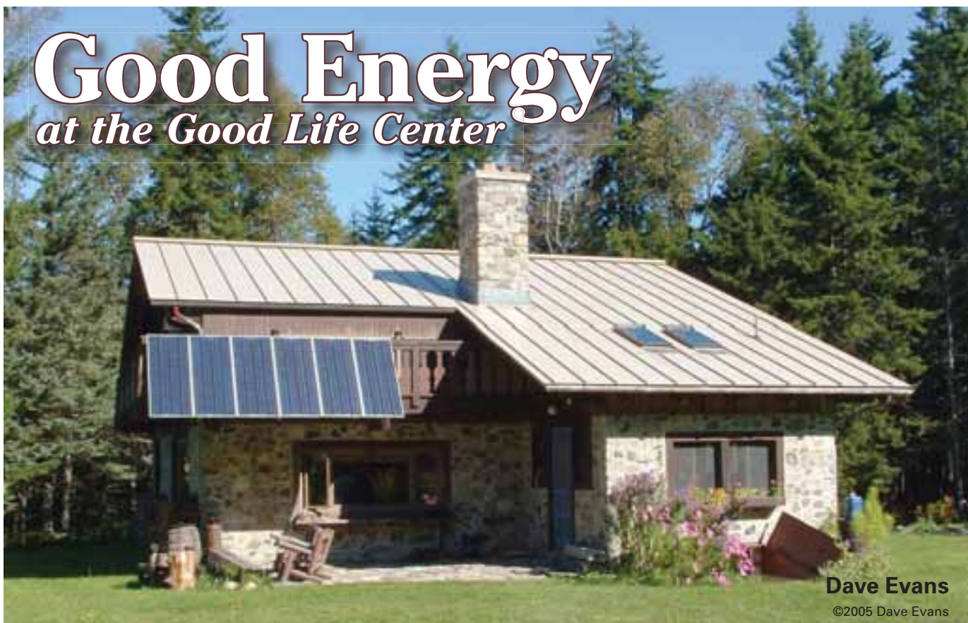
The solar-electric system helps demonstrate the Good Life Center's commitment to sustainable living.
