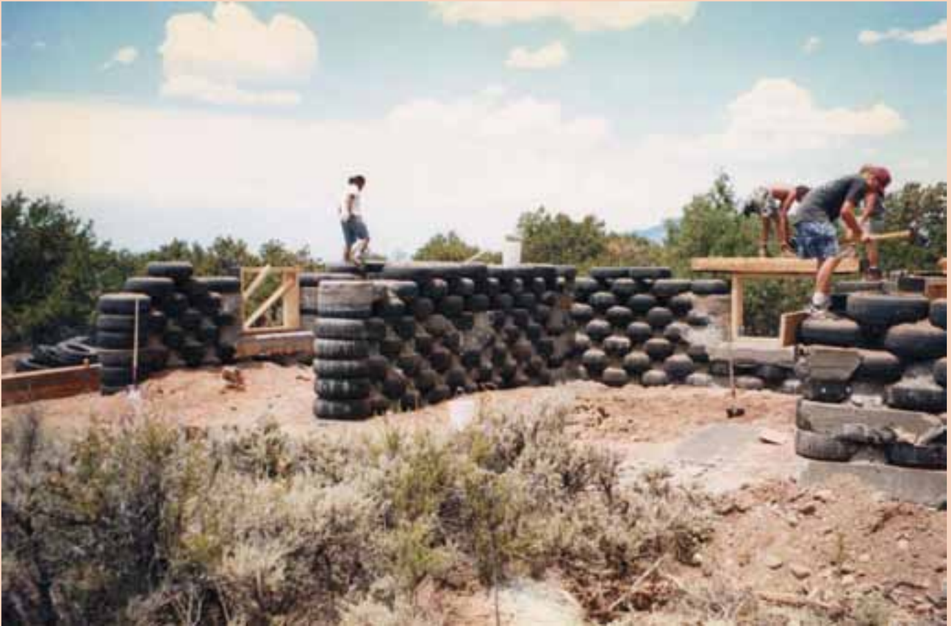
Almost 500 used car tires, filled with compacted earth, were used in the construction of the home's walls.
