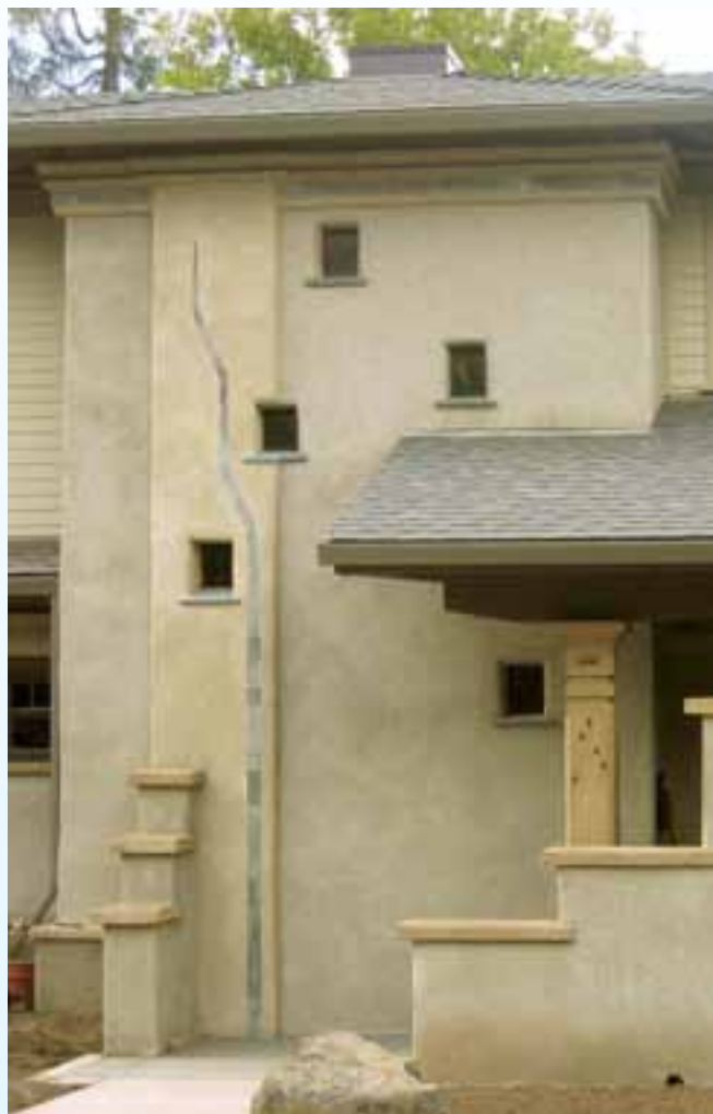
In hot, arid climates, high thermal mass like adobe walls temper heat fluctuations. Small windows on the south wall reduce heat gain.
