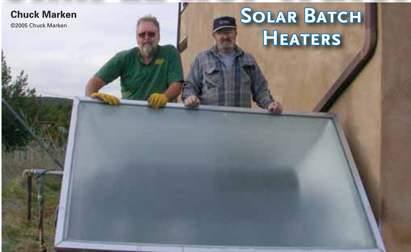
Author Chuck Marken and Don Keefe of AAA Solar rebuilt and reinstalled this Cornell batch heater.
