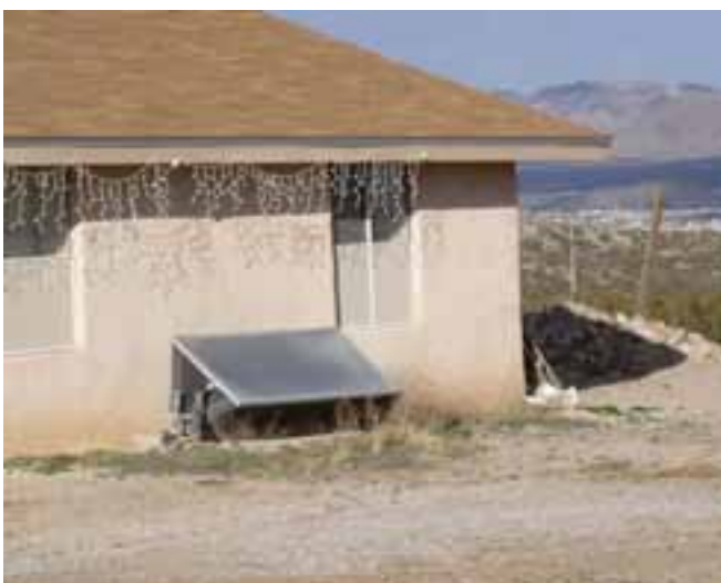
Batch solar water heater in Santa Theresa, New Mexico.
