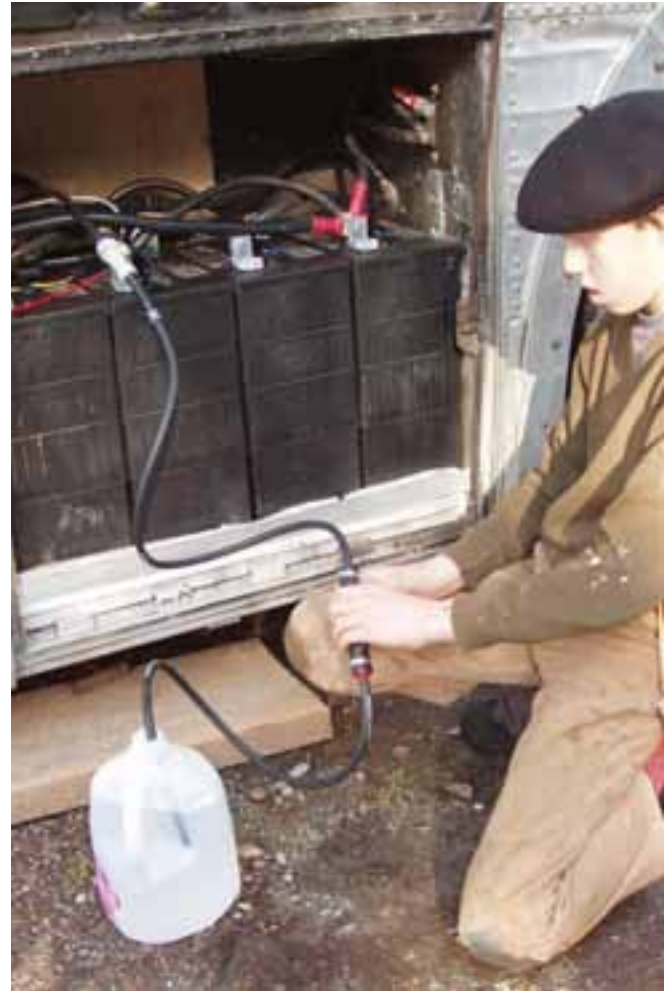
Zander Woofenden filling the bus battery bank with the Pro-Fill battery watering system.
