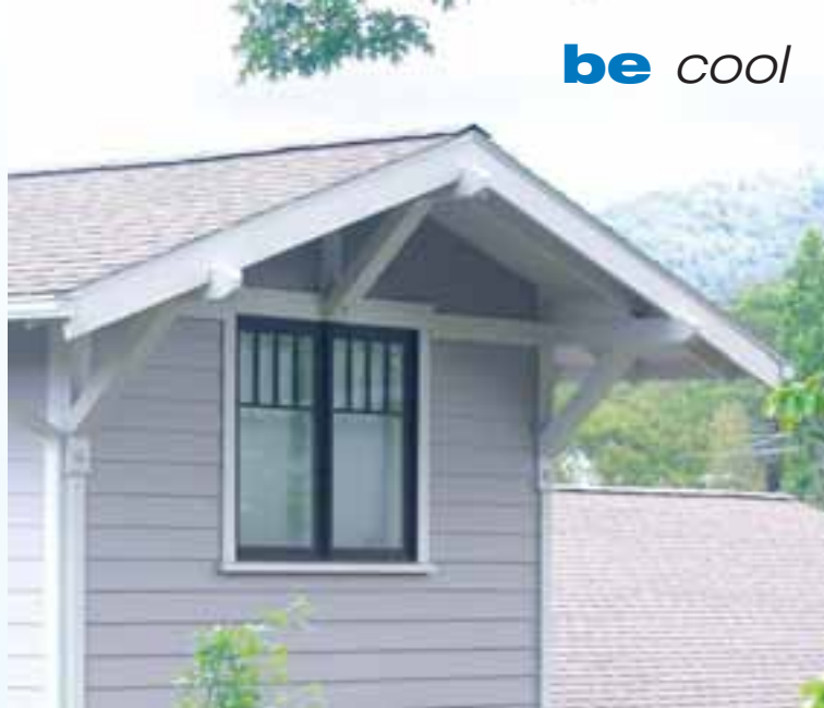
Properly sized overhangs shade windows from the high summer sun, but allow the low winter sun to enter.
