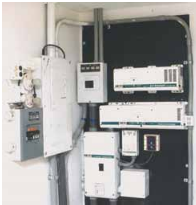
In the power room, hydro and solar power converge. When the batteries are full, excess hydro or solar electricity is used to heat domestic water.
